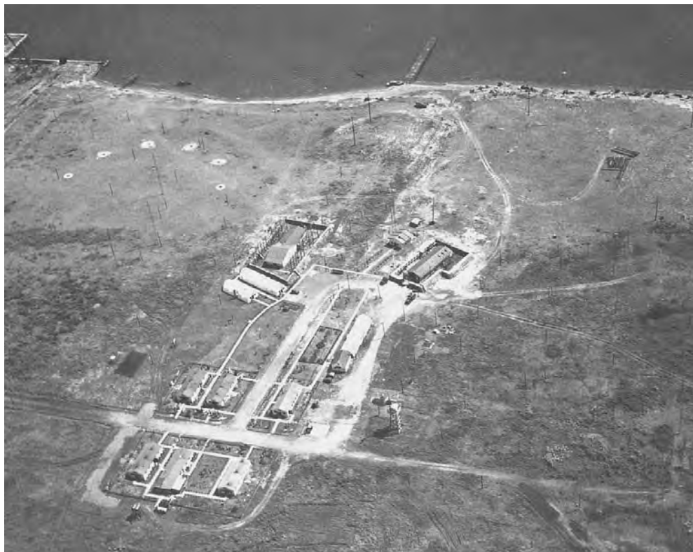
Aerial view of a long distance radiotelephone receiving site in Japan
